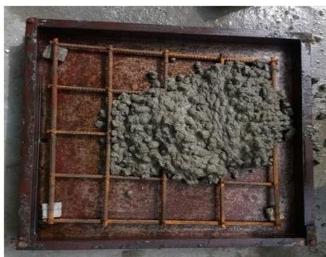
Figure5.1: Slab mould with reinforcement
