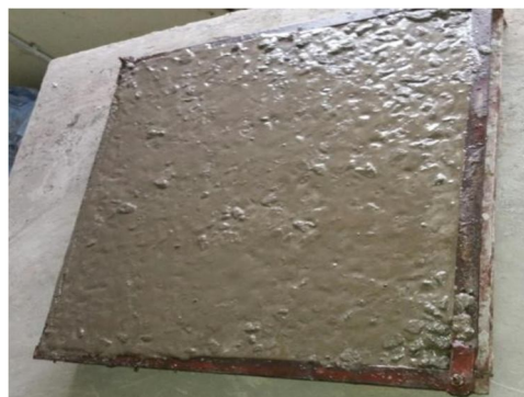
Figure 5.2: Slab mould filled with concrete
