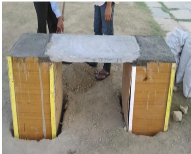
Fig 5 Pouring of concrete and slab in wooden framework.
