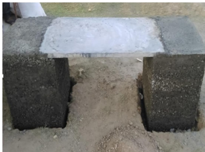
Fig 6. After completion of the construction
