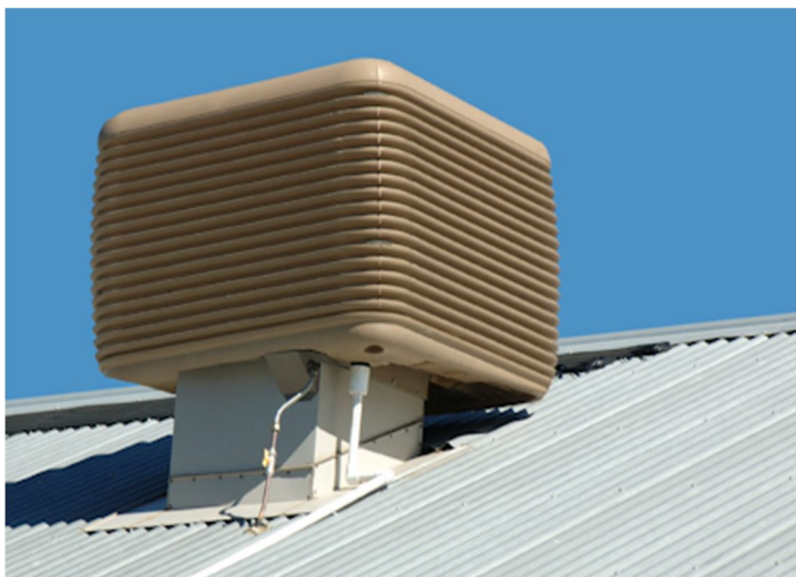
Fig. 1 Fresh Air Unit
