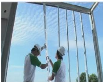
Fig. 3 Fixing steel frame in position.
