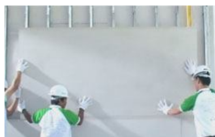
Fig. 6 Mounting of board on other side of frame.
