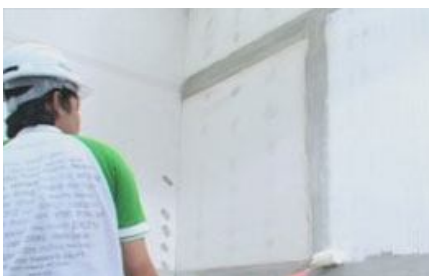
Fig. 8 Finishing of joints with Shera PU sealant.
