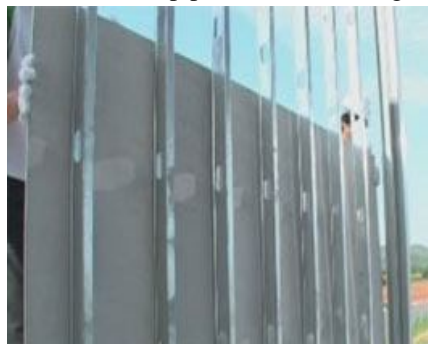
Fig. 4 Mounting 8mm SHERA board on one side
