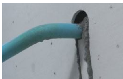
Fig. 7 Pumping light weight concrete from top
