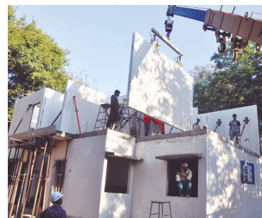
Fig. 2 Installation of a GFRG panel (Source : BMTPC )
