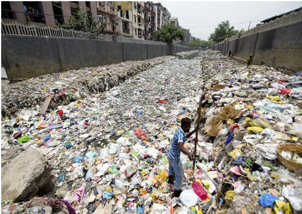
Fig. 1 An open drain clogged due to plastic waste
