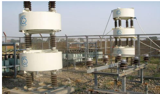
Fig: Air Core Dry Type Reactor
