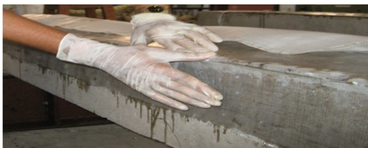
Fig. 6 Fixing of GFRP sheet on the beam
