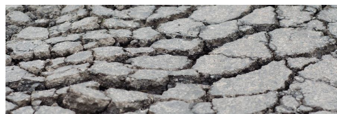
Fig 1.1 Shrinkage Cracks
