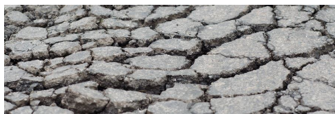
Fig 1.1 Shrinkage Cracks
