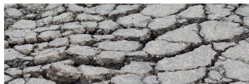
Fig 1.1 Shrinkage Cracks
