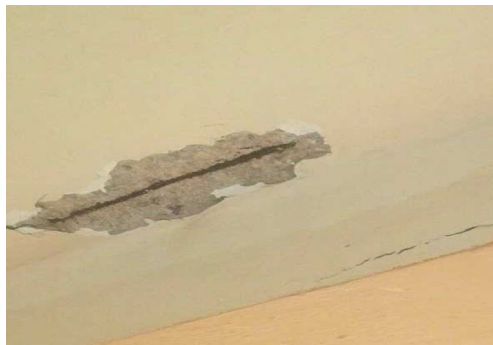
Fig 3: Spalling of Concrete and corrosion of reinforcing bars Fig 4: Moisture Ingress
