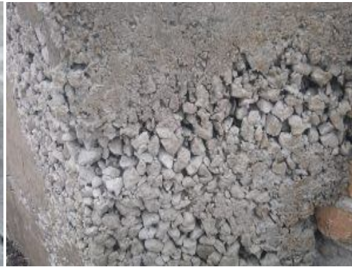
Fig 1: Cracks on concrete surface Fig 2: Honeycombing
