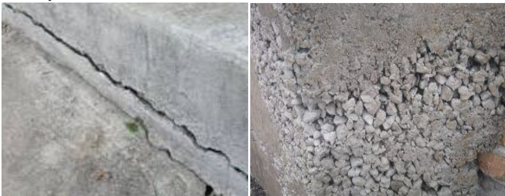
Fig 1: Cracks on concrete surface Fig 2: Honeycombing
