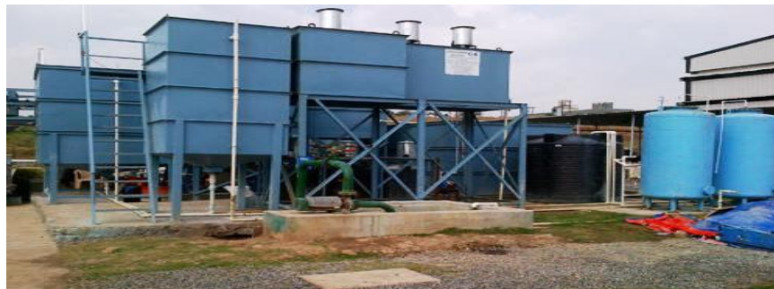
Fig 6 Waste Water Treatment Plant
