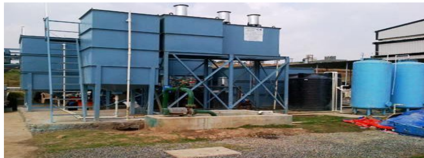
Fig 6 Waste Water Treatment Plant
