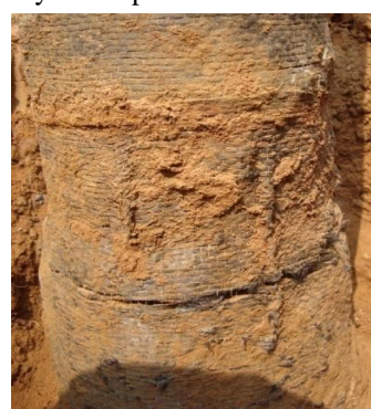
PFRP confined pile
