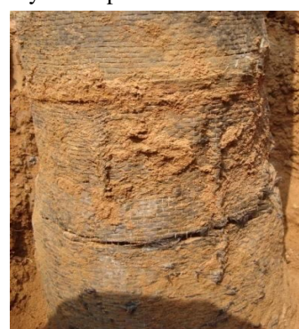
PFRP confined pile
