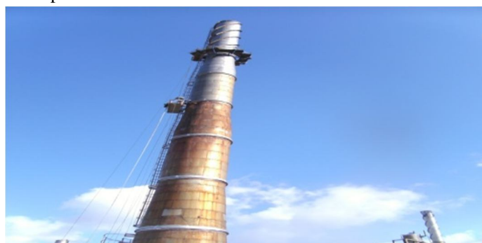
Figure -1: Industrial Steel Chimney (Ref: Anonymus)
