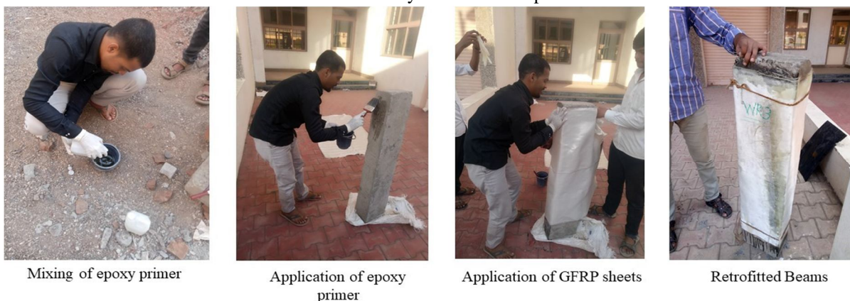
Fig.4. Retrofitting of RC beam by using GFRP
