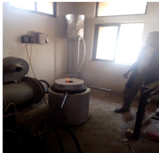
Fig. IV Furnace being heated.
