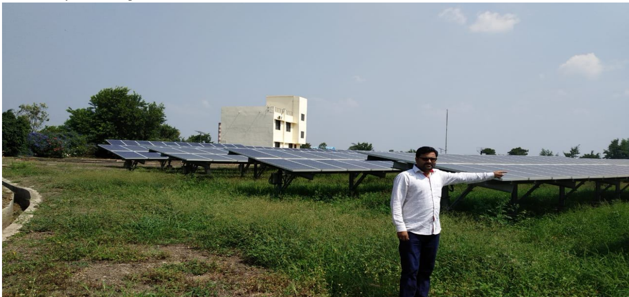
Fig. 1 Visit to solar power plant of 1 MW power generation capacity.
