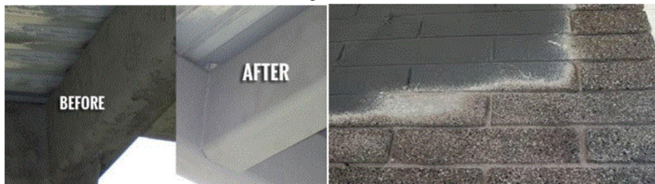
Fig.9 Comparison Between Surfaces Before and After Sandblasting[7]
