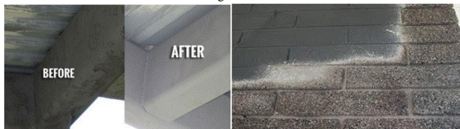
Fig.9 Comparison Between Surfaces Before and After Sandblasting[7]
