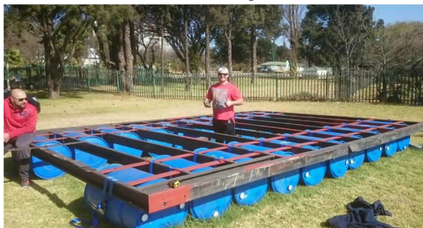
Fig 2: Drum Pontoon based foundation
