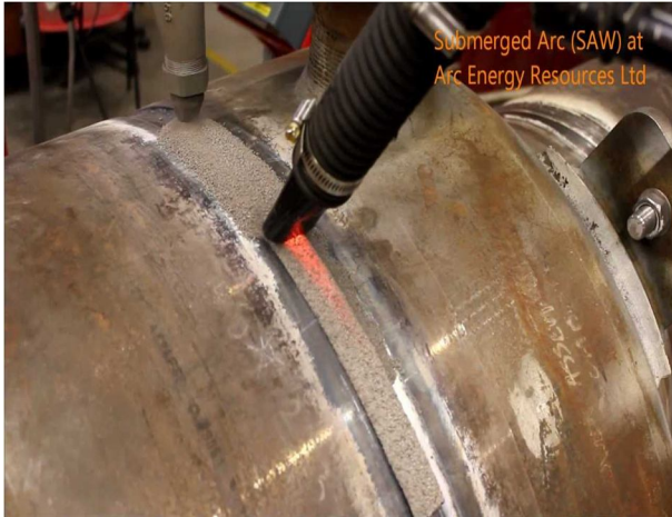
Figure.4.1 Welding Of Cylinder
