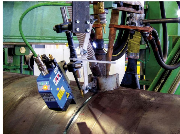
Figure.4.2 Welding Of Pipe
