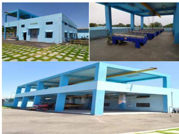
Fig.9. View of Centrifuge unit
