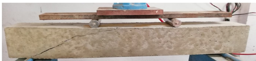
Figure 6 Cracked pattern of two layer geogrid reinforced beam
