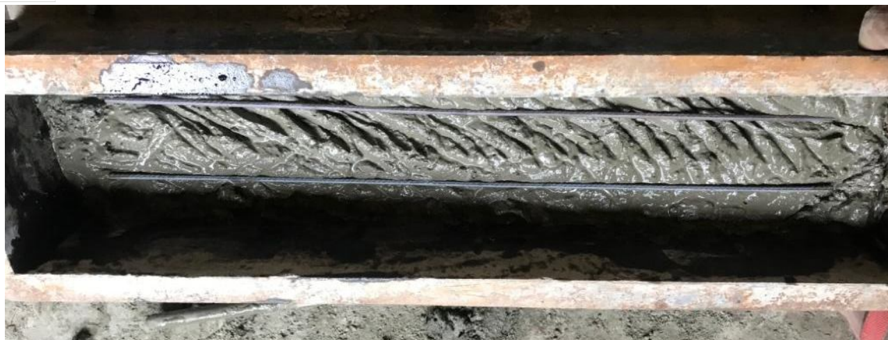
Fig.28 Placing rebars for reinforcement
