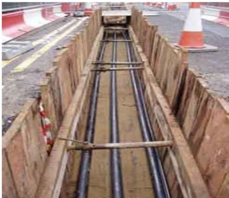
Fig 2: Underground cable laying
