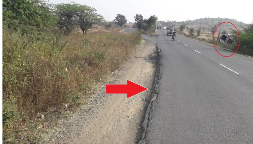
Figure 7:-Improper shoulders at ghat section between Chhegoan Makhan (Kherda village) To Roshiya
