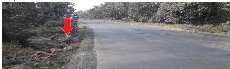
Figure 9:-Formation width is eroded due to excess rainfall.
