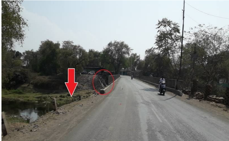
Figure 15:- Guardrails are broken at Sanawad Bridge
