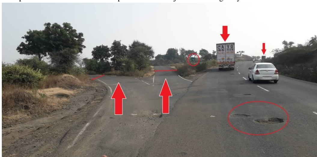
Figure 6:- Heavy trucks do not follow diversion road and rule & regulations and potholes at ghat section between Chhegaon Makhan (Kherda village) To Roshiya
