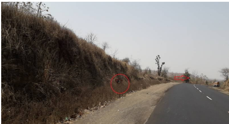
Figure 10:-Sign board direction changed due to wind force or hit by any vehicle
