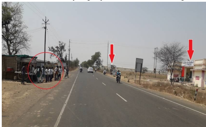
Figure 4:- No signs boards, road markings and speed breaker In Front of Govt.School Takali Mori (Chhegaon Devi)
