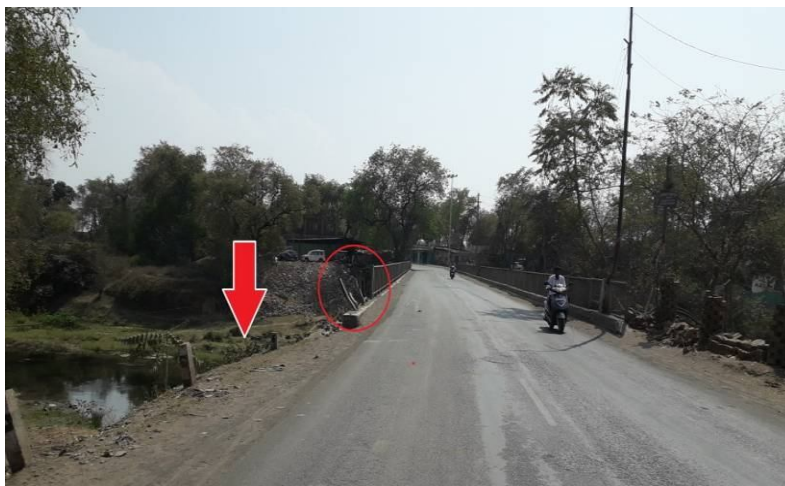
Figure 15:- Guardrails are broken at Sanawad Bridge
