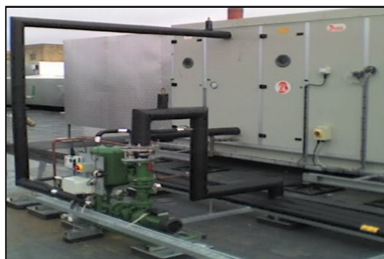
Fig.2: Run-around Coil
