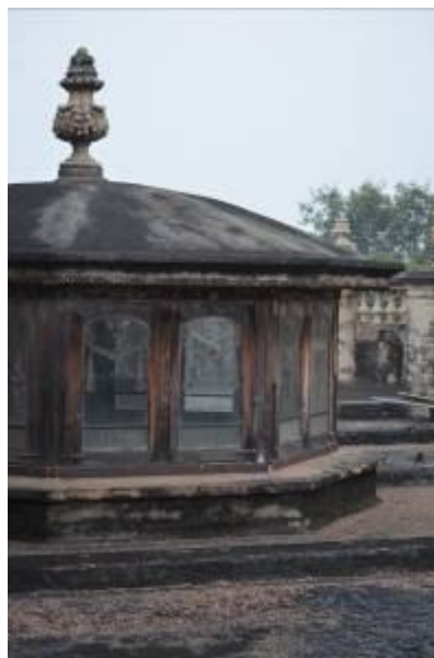
Fig. 5 The Skylight at the roof level
