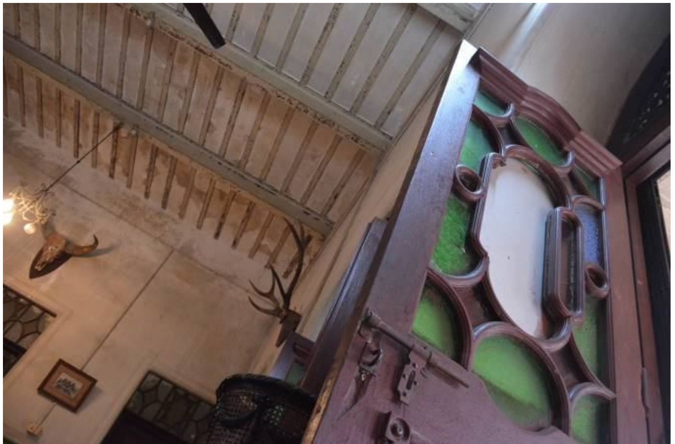
Fig. 26 Iron Girder Ceiling and Wooden Door
