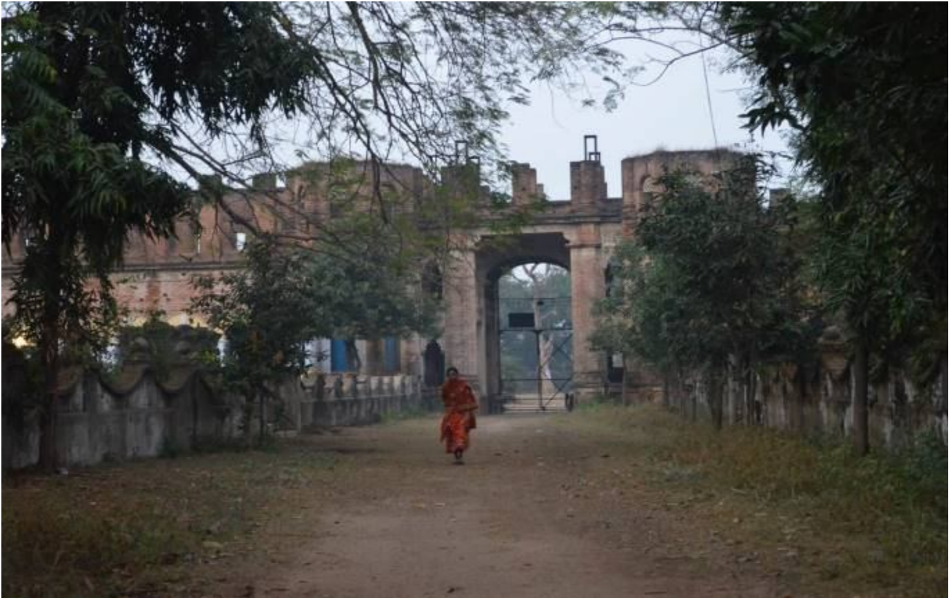
Fig. 20 Boundary Wall and Entrance Gate
