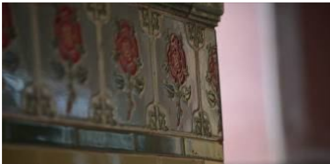
Fig. 36 Inlay work on the Wall
