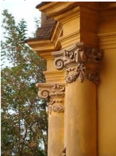
Fig. 4 The Composite Columns and Cornice
