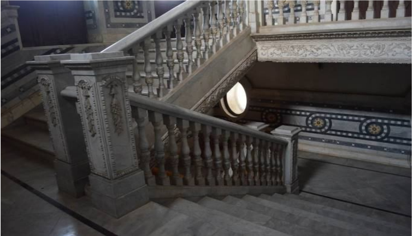
Fig. 27 Intricate Railing and Marble flooring work in the Staircase
