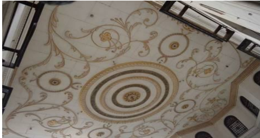
Fig. 35 The Gold Gilding work on the Ceiling
