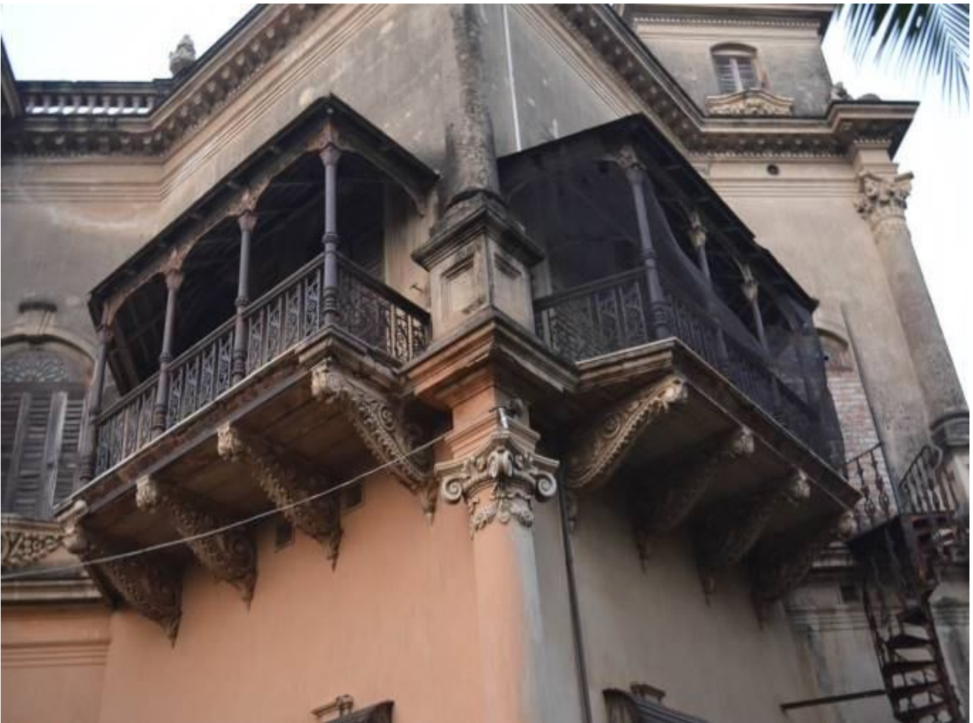
Fig. 33 Balconies at First Floor Level
