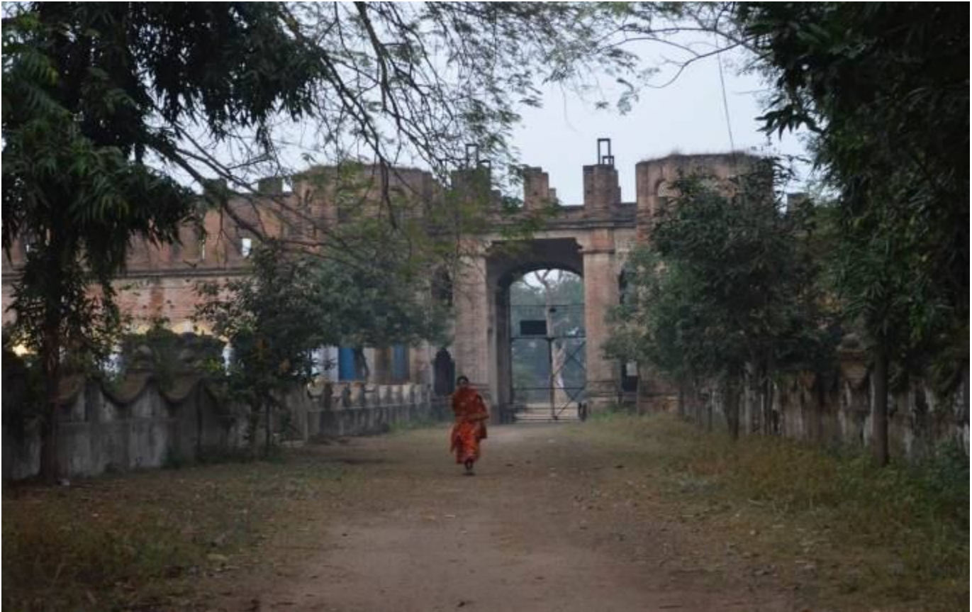
Fig. 20 Boundary Wall and Entrance Gate
