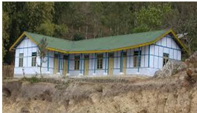
Fig 3: Ikra type housing [24]
