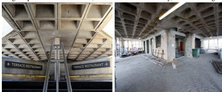
Fig. 1: Typical examples of waffle slab
