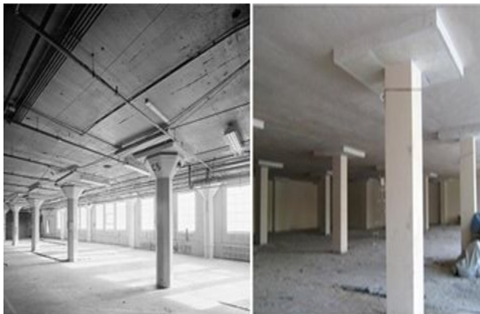
Fig. 3: Typical examples of flat slab
