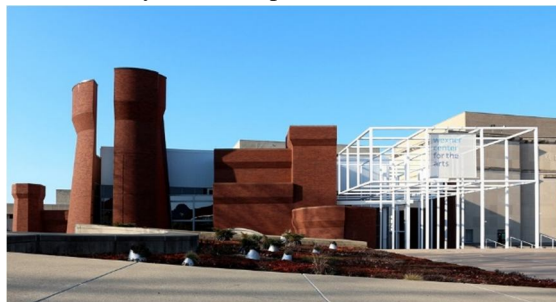
Figure 3: Wexner Center for the Arts (Web Urbanist, 2011)
