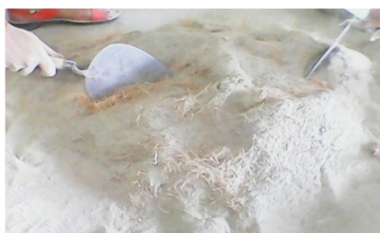
Fig 1. Mixing of Fibres with cement
