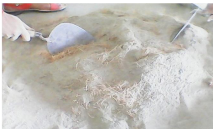
Fig 1. Mixing of Fibres with cement
