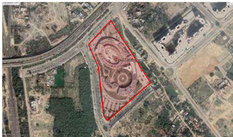
Figure 11-Satellite images of the Avadh Shilpgram Located in Lucknow (Image Courtesy of Google Earth)
