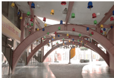
Figure 16-View Shows the Beam of M.S.
