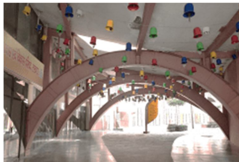
Figure 16-View Shows the Beam of M.S.
