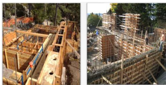
Fig. 1. Wooden Formwork
