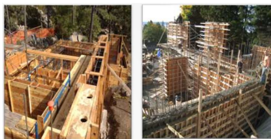
Fig. 1. Wooden Formwork
