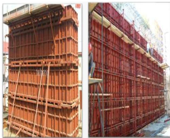
Fig. 2. Steel Formwork
