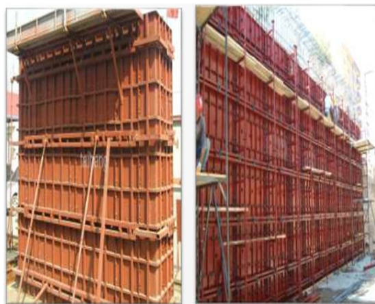
Fig. 2. Steel Formwork
