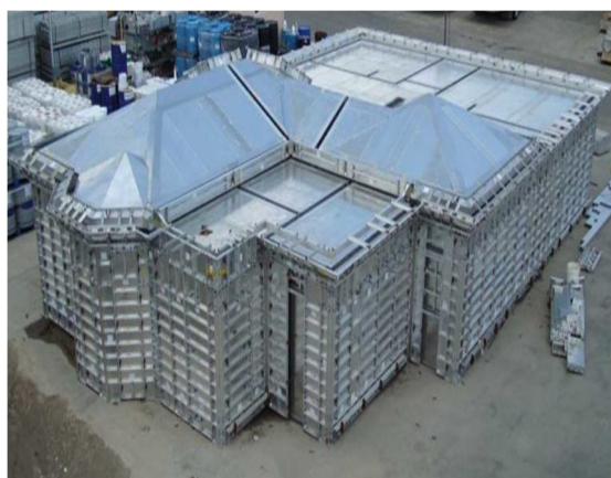
Fig. 3. MIVAN Formwork System
