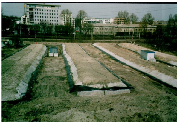
Fig. 3. View of the remediation facilities with the piles, service containers and bioreactors
