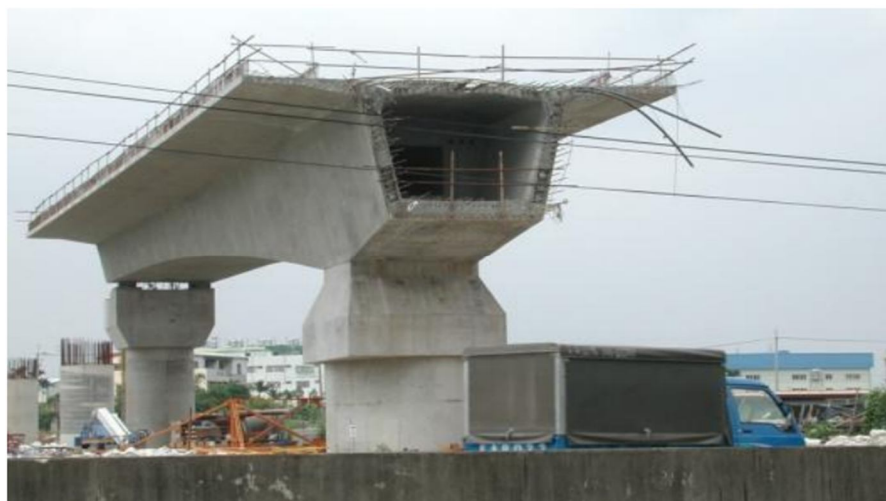
Figure 1: Box Girder Bridge
