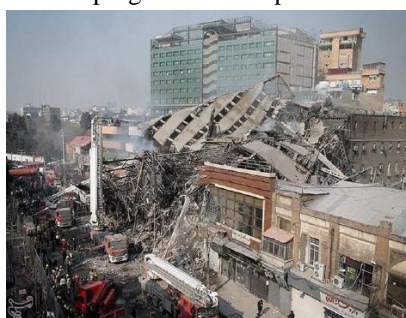
Fig 2 Plasco Building Progressive Collapse
