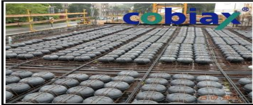
Fig. 2 Flat slab or Voided slab
