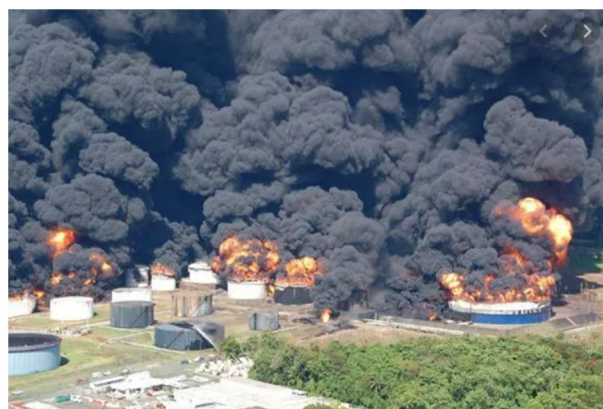
Figure 2: Industrial disaster due to gas leakage.
