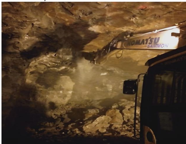
Figure Scaling & Trimming
