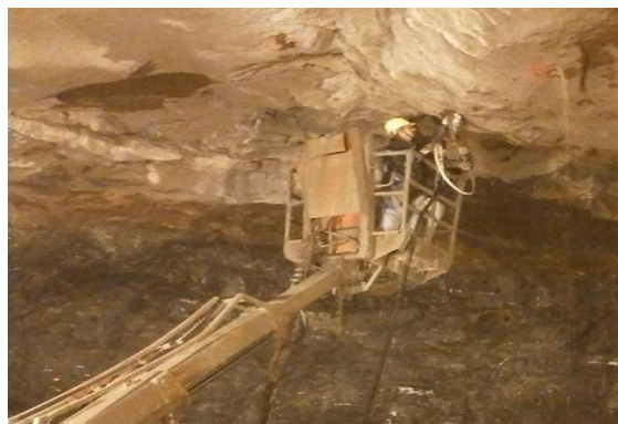
Figure. Rock bolting
