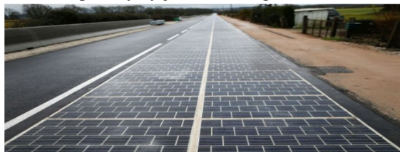
Fig 1(a) solar road
