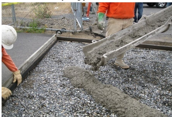
Figure 6. Recycled Aggregate Concrete For Within Site Recycling
