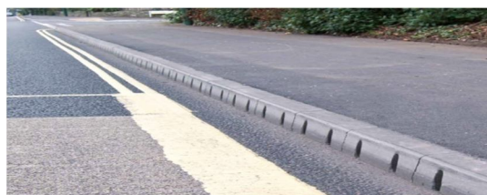
Figure 2. Recycled Aggregate as Road Kerb
