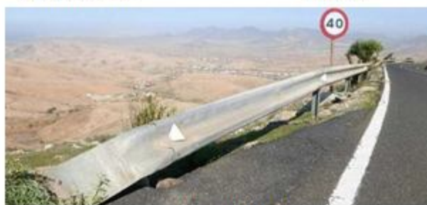
Damaged Steel barrier
