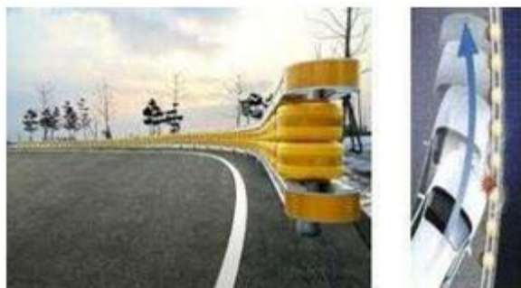
Figure 1.1: Rolling Barriers at the Roadside and vehicle collision
