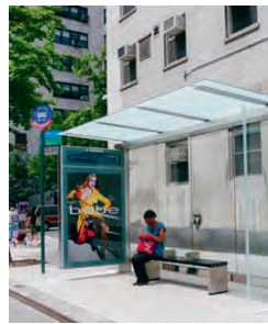
Fig.5: Bus stop shelter
