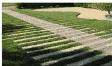
Fig. 32 A. Porous pavers to increase water percolation
