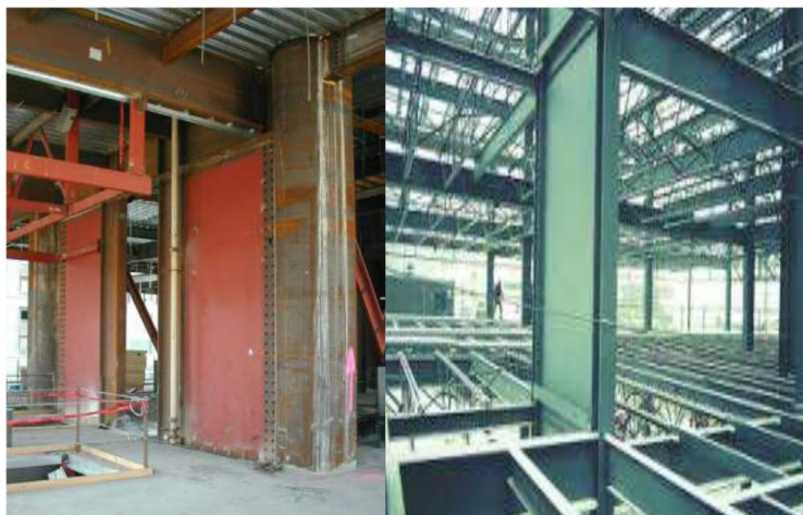
Fig. Steel Plated shear wall.
