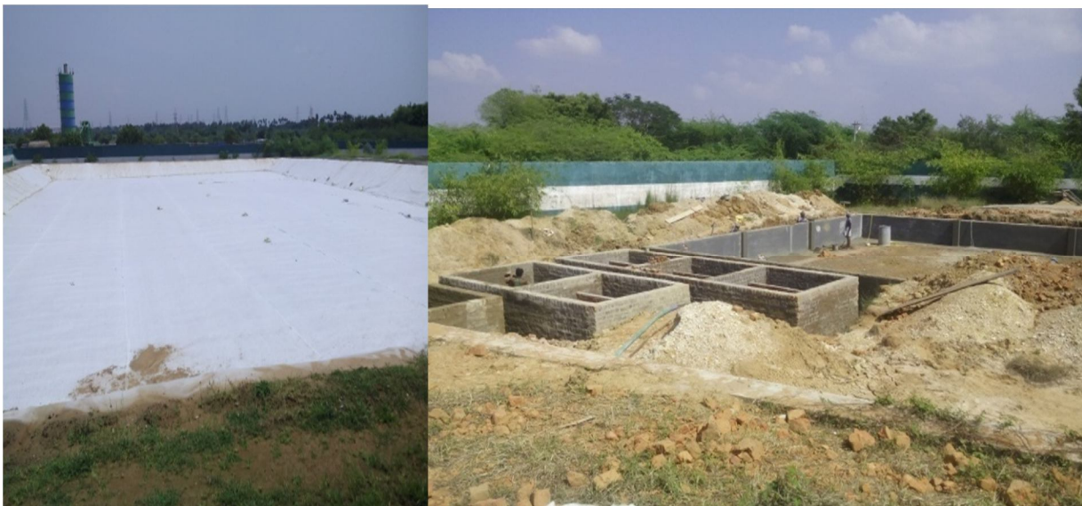
Figure 3.10 Scientific Landfill and Tanks
