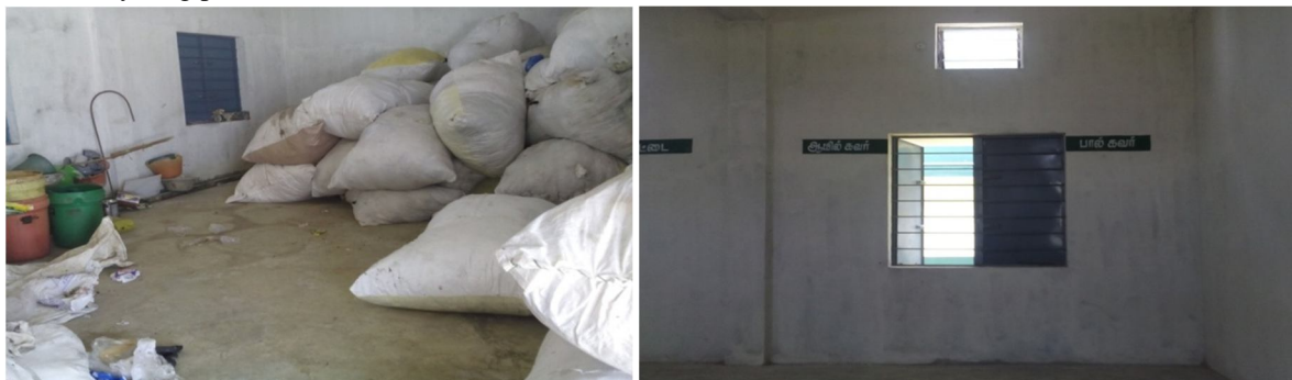
Figure 3.9 Storage Rooms For Recyclable Materials
