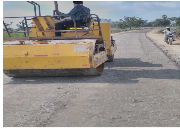
Fig. 6 WMM rolling by vibratory drum roller
