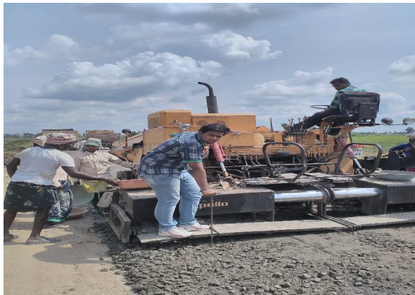
Fig. 5 WMM laying by paver & author checking thickness
