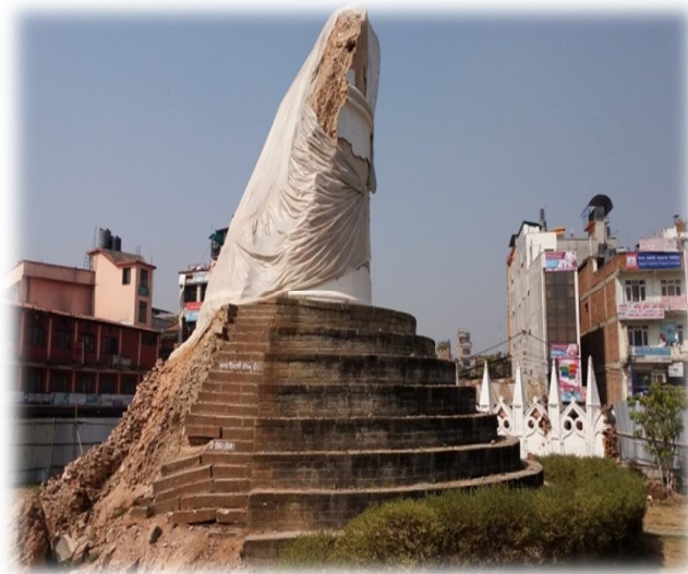
Figure 1: damaged dharahara tower, kathmandu
