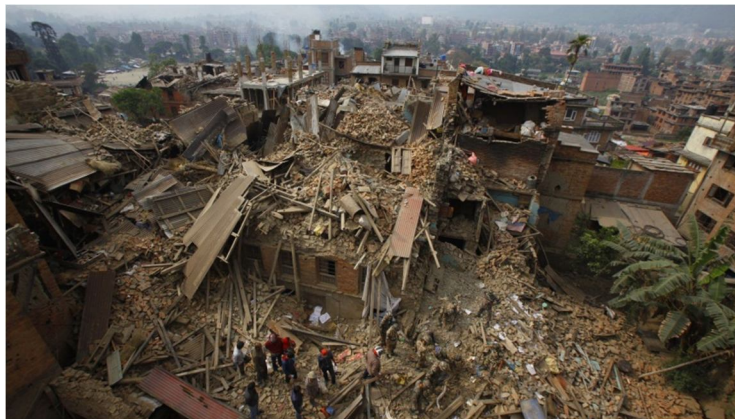
Figure 3: total house collapsed
