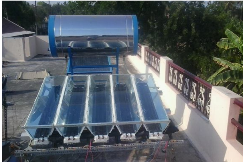
Fig no: 3 Construction of v-trough
