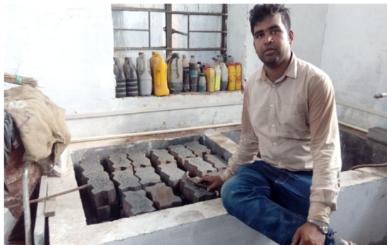
Curing of paver block
