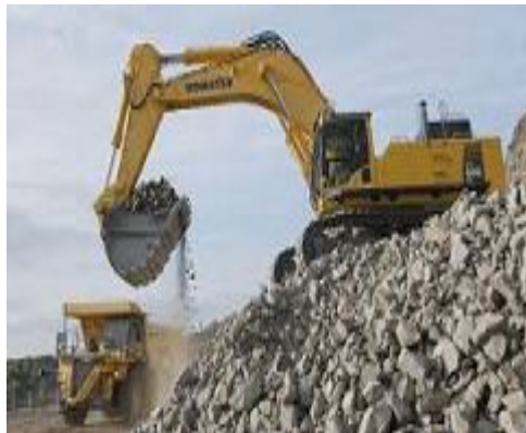
Fig: Hydraulic excavator
