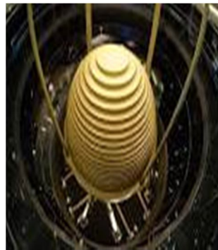
Fig: 4 Tuned mass Damper
